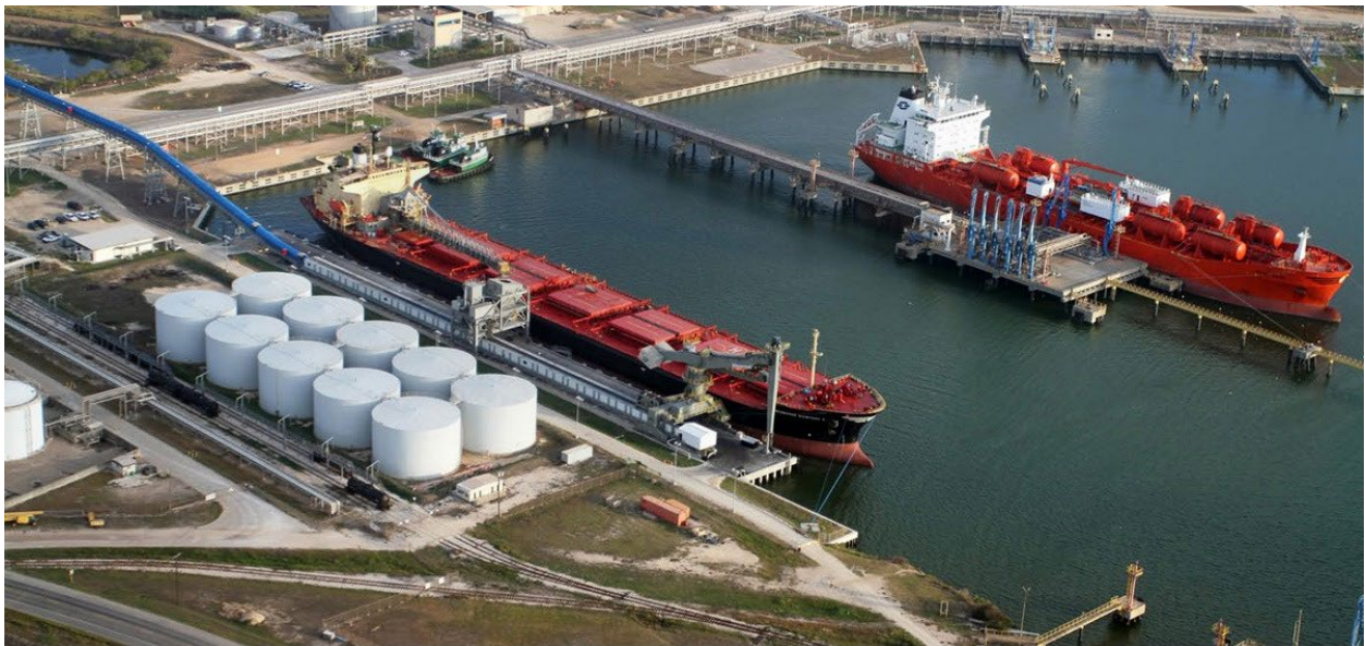
Figure 1-4: View of CPA Docks at Point Comfort Turning Basin (2)
